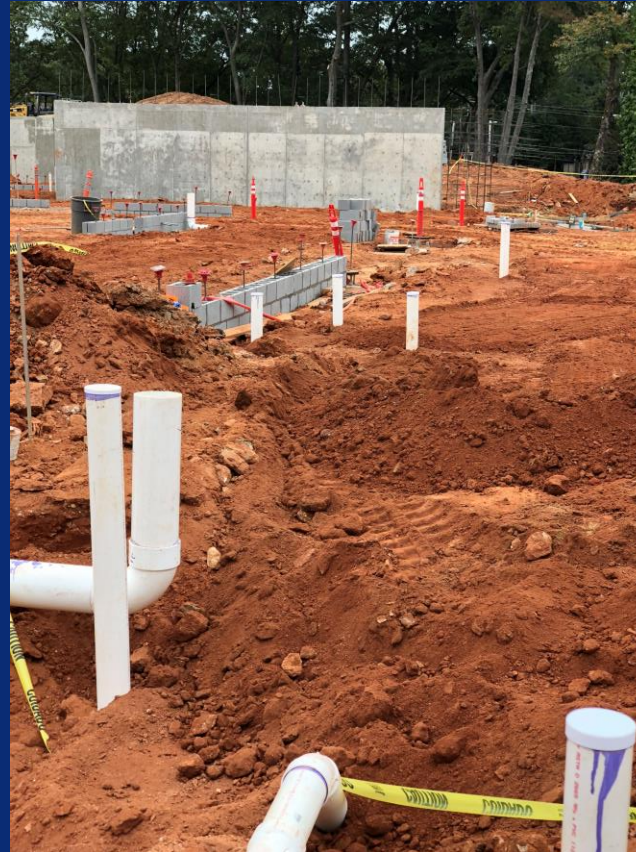
All lower level underground sanitary lines installed and inspected
