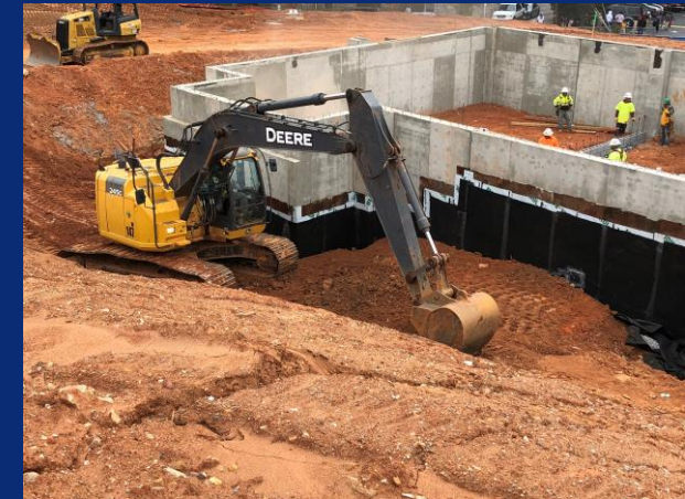
Backfilling along northeast corner near elevator
