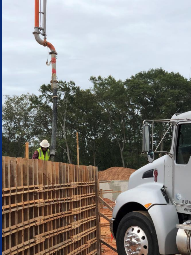
Retaining wall at northwest corner of gymnasium being poured
